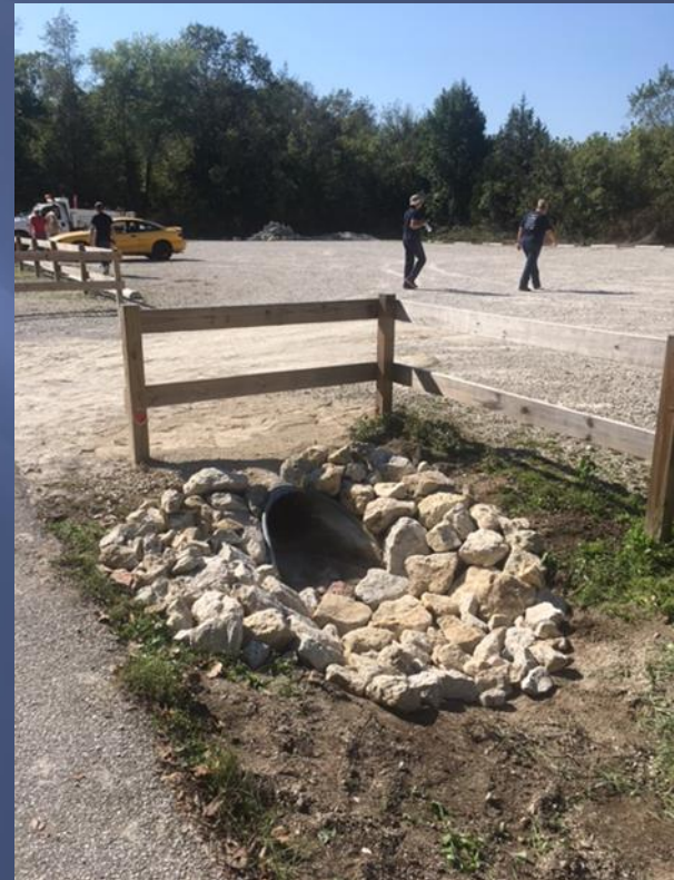
Lining the culverts to facilitate drainage
