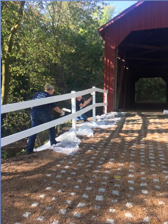
Painting the approach rails
